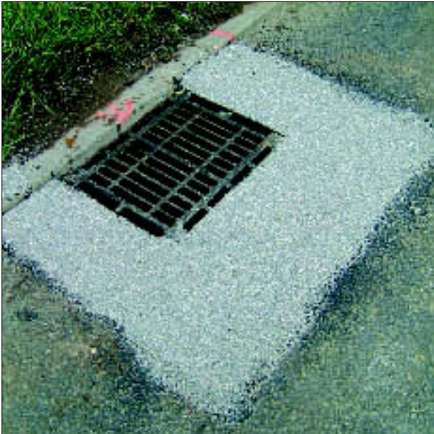
Figure 5 Anti-slip aggregate applied
