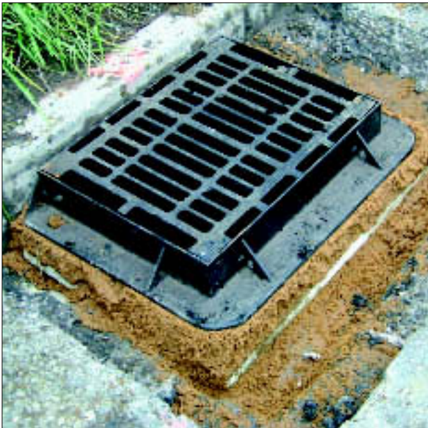
Figure 2 Frame bedded on Ironmaster Mortar P
