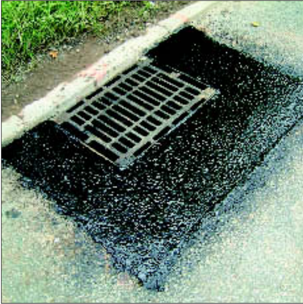
Figure 5 Anti-slip aggregate applied
