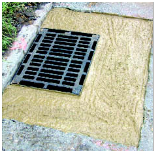
Figure 3 Ironmaster infill applied
