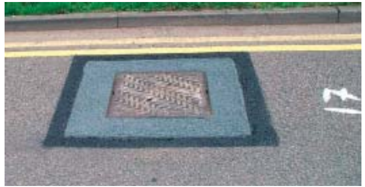
Working flat out: Glasgow monitored a total of six repair systems. The above show ironwork before (left) and after with Ironmaster
