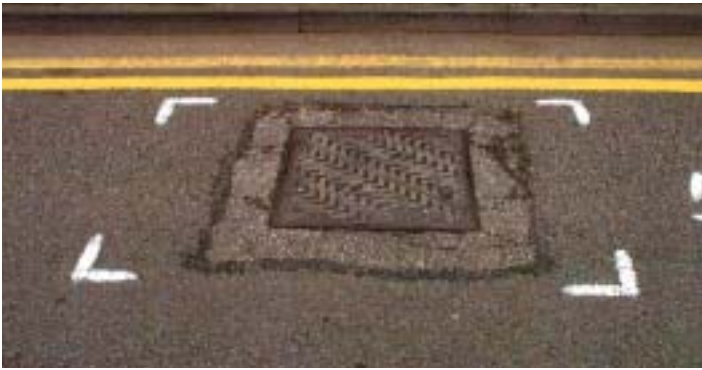
Working flat out: Glasgow monitored a total of six repair systems. The above show ironwork before (left) and after with Ironmaster
