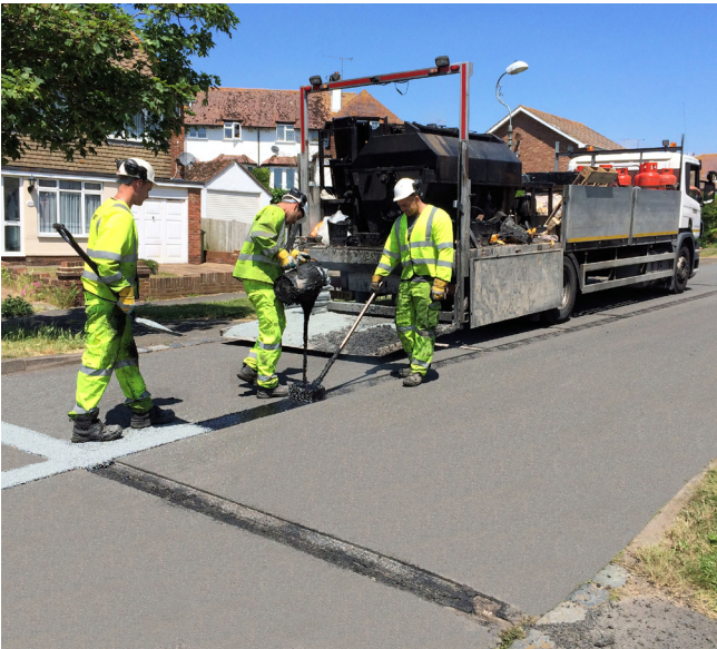
Estate Road installation in East Sussex. Repairing cracks in thin asphalt overlay on a concrete base.
