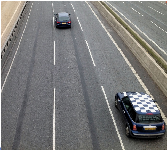
M4 Motorway Bristol. Seam joints repaired as part of Smart Motorway Scheme.
