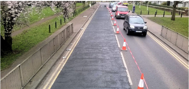
Treatment of complete lane
