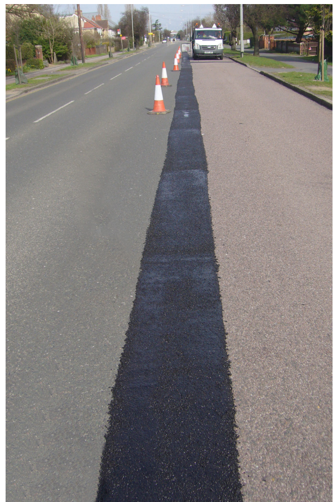
Repaired asphalt seam joint
